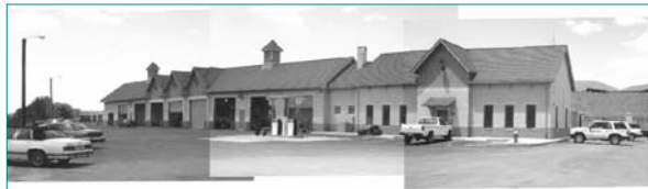
The garage maintenance facility is attached to the satellite office facility for the Department. The industrial tone of the building was lightened with the use of cupolas, asphalt shingles and wood windows.
