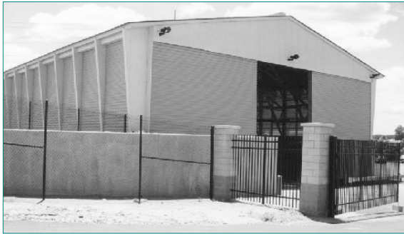
Public Works salt storage building features high, clear-span wood trusses.
