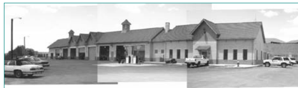
The garage maintenance facility is attached to the satellite office facility for the Department. The industrial tone of the building was lightened with the use of cupolas, asphalt shingles and wood windows.
