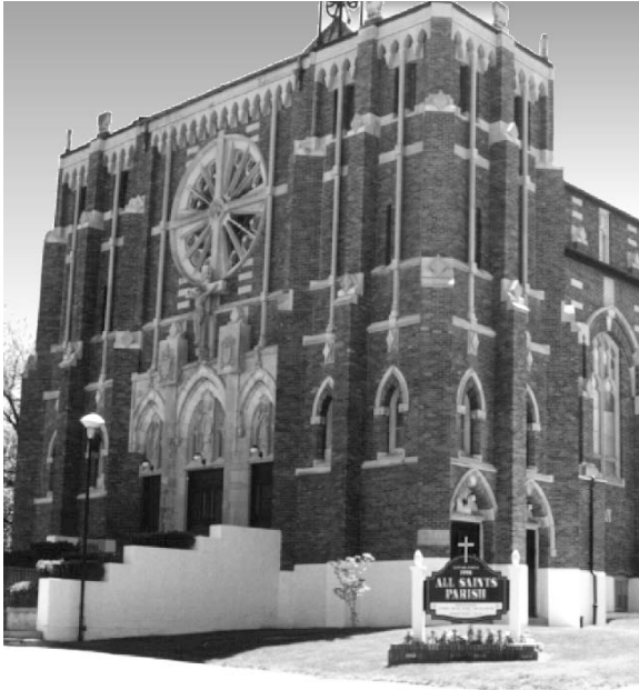
All Saints Parish in Haverhill, Massachusetts received renovations to two of their buildings adjacent to their Church. The work was completed for the local church under the direction of the Archdiocese of Boston.
